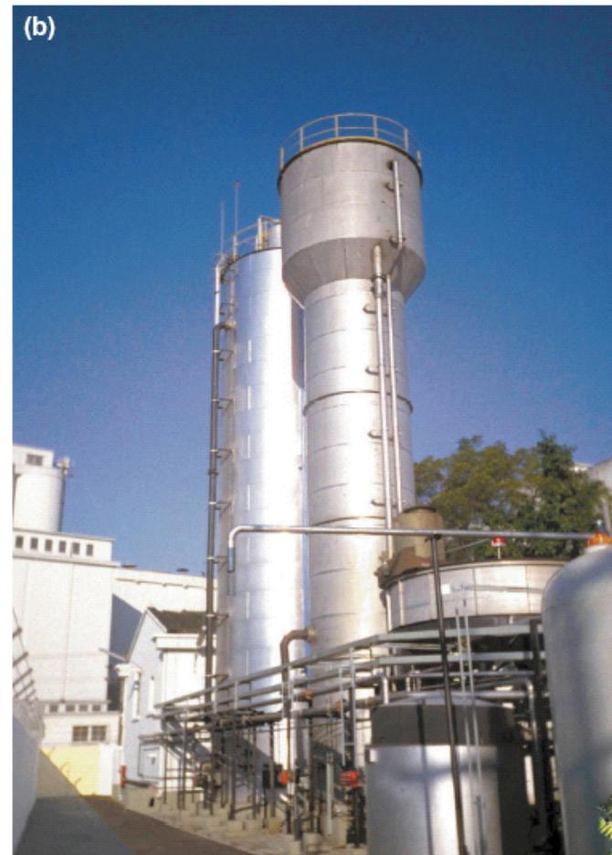
**Expanded Granular Sludge Bed (EGSB) reactors**
